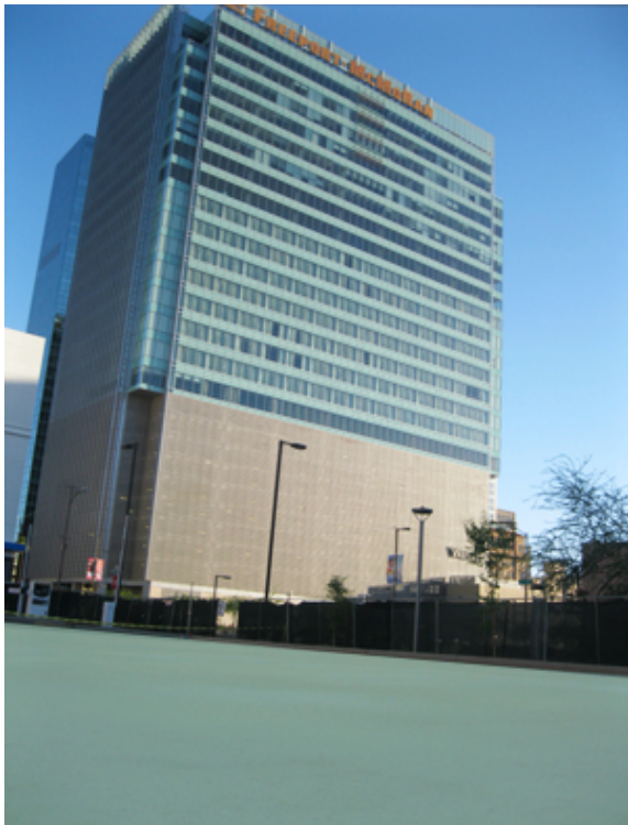
View of Westin Hotel from “Cool Pavement”
